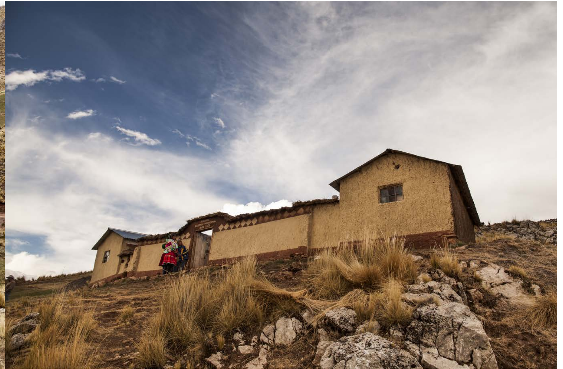
➔ A house with a future. The new healthy home owned by Ricardina Mamani and her husband Antonio Picho is the axis around which the family has built a sustainable life project.
